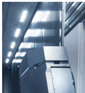
LED lighting in the working area.
